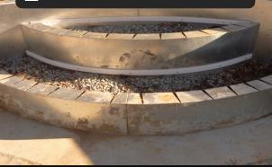
Backfill with gravel, stone or sand. Leave 2" to accommodate finishing material. Face-mount liner track 1/4" higher than tread height.
