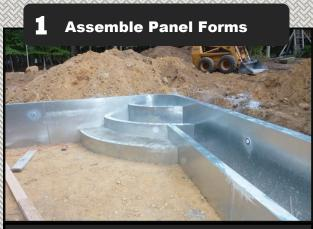
Fasten panel forms to perimeter panels using prepunched bolt holes. Secure forms with drive stakes. Pour a 6" footer inside each cavity.
