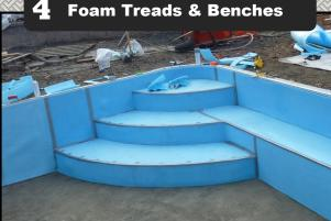
Tape steel-cement seams. Foam tops of treads & benches with 1/4" high density material. Optional 1/8" wall foam can be installed on risers & walls.
