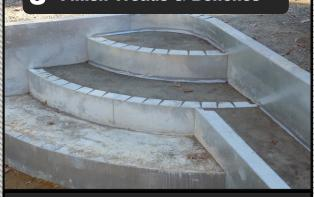
Cover liner track with tape. Finish off tops of treads and benches with concrete or grout mix.
